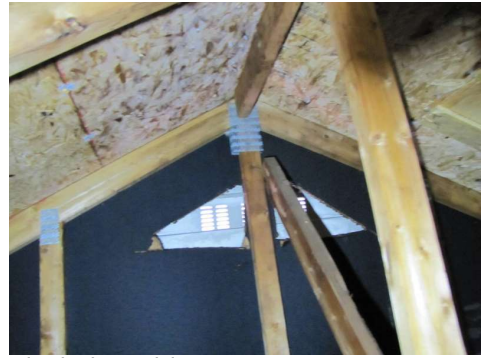
Block the gable vent
