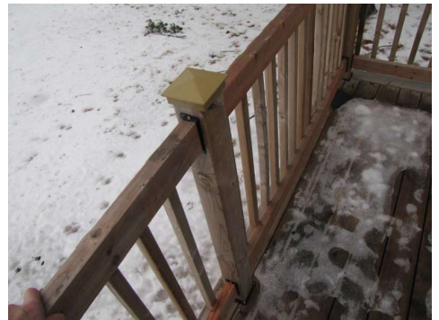
Back balcony the railing was loose
