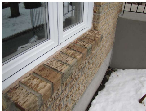
Cracks between the bricks are visible allowing water infiltration into the wall below
