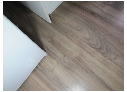
Under the fridge area
