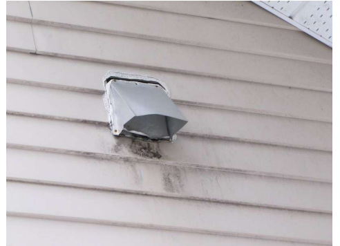
It appears the the vent is not functioning properly.
