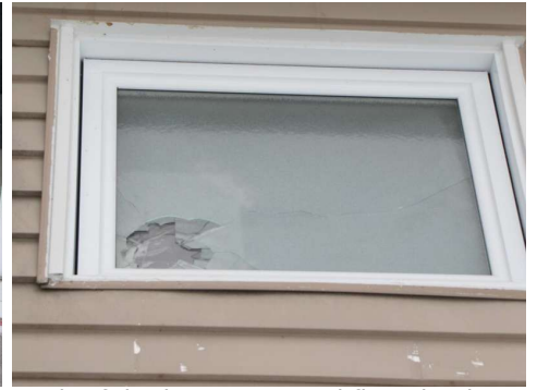
Back of the house second floor broken glass
